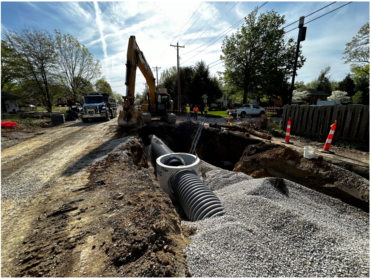
(BBI installation of 36" storm sewer and Manhole Str. #136 along Walnut Street.)
