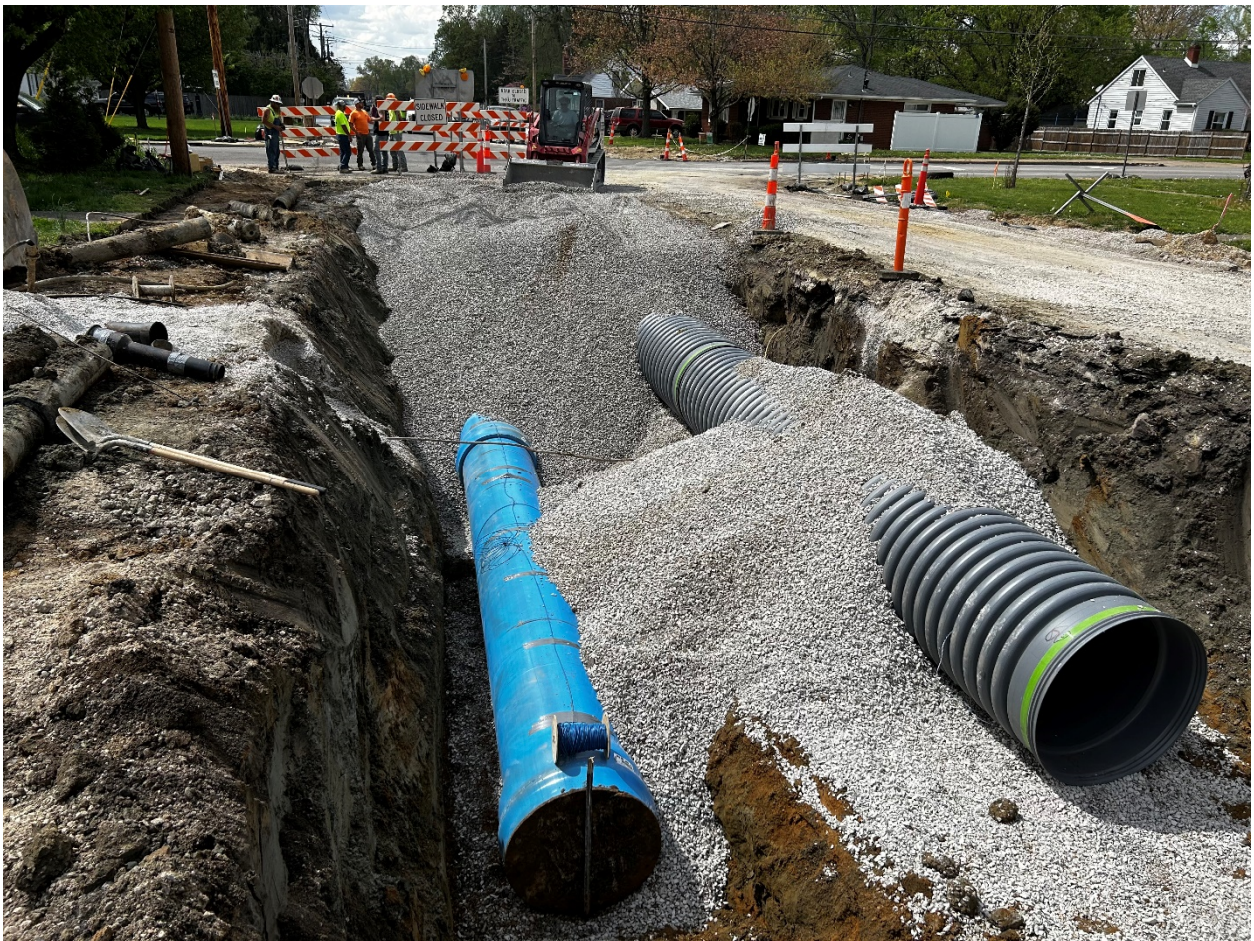
(BBI installing both 30" force main and 36" storm sewer along Walnut Street.)
