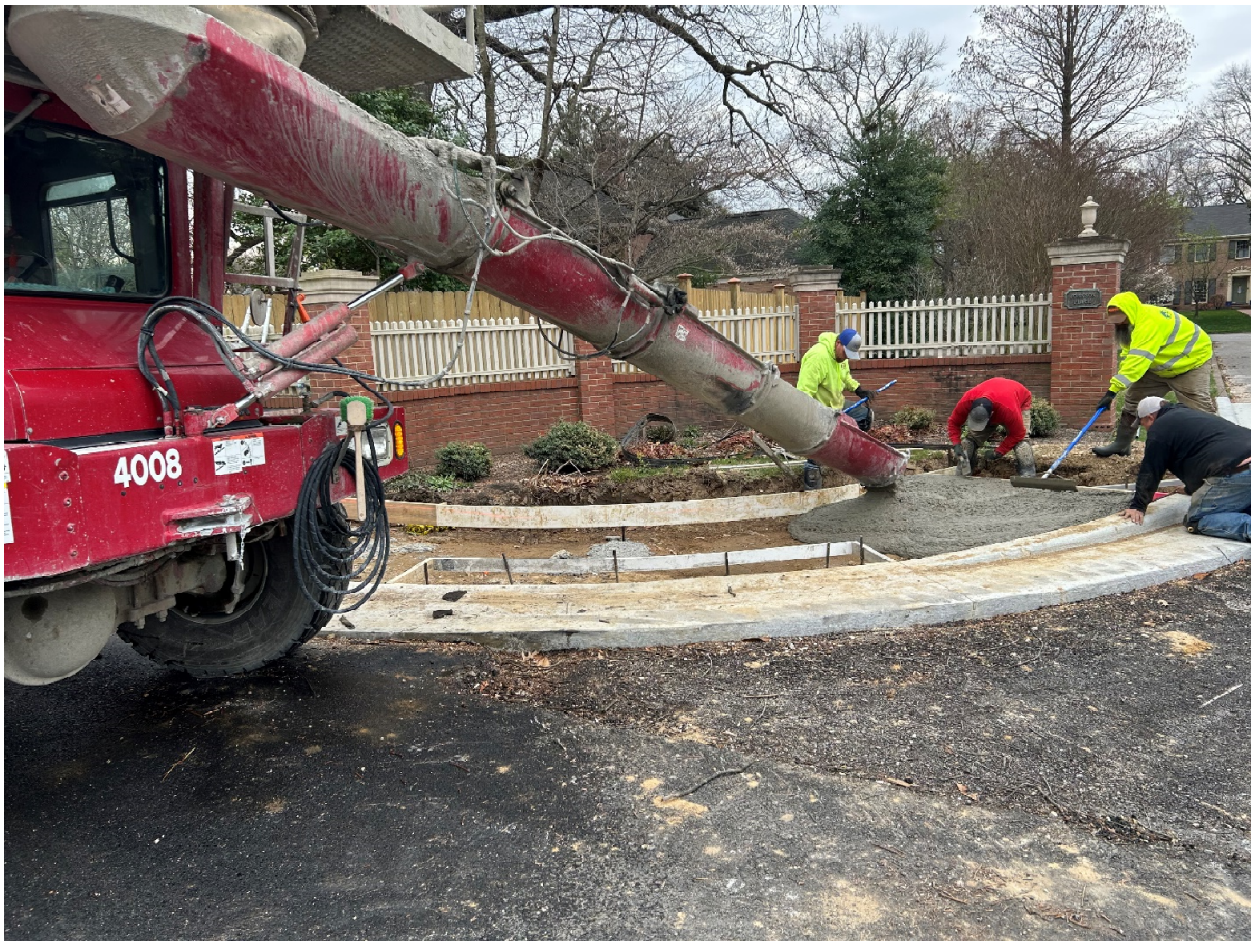
(BBI pouring curb ramp at the southeast corner of Johnson Place and Walnut Street.)
