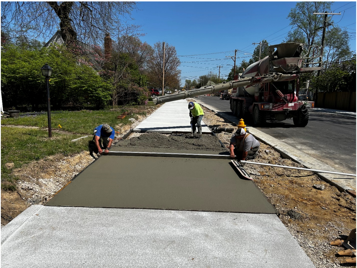
(BBI pouring multi-use trail along north side of Walnut Street.)
