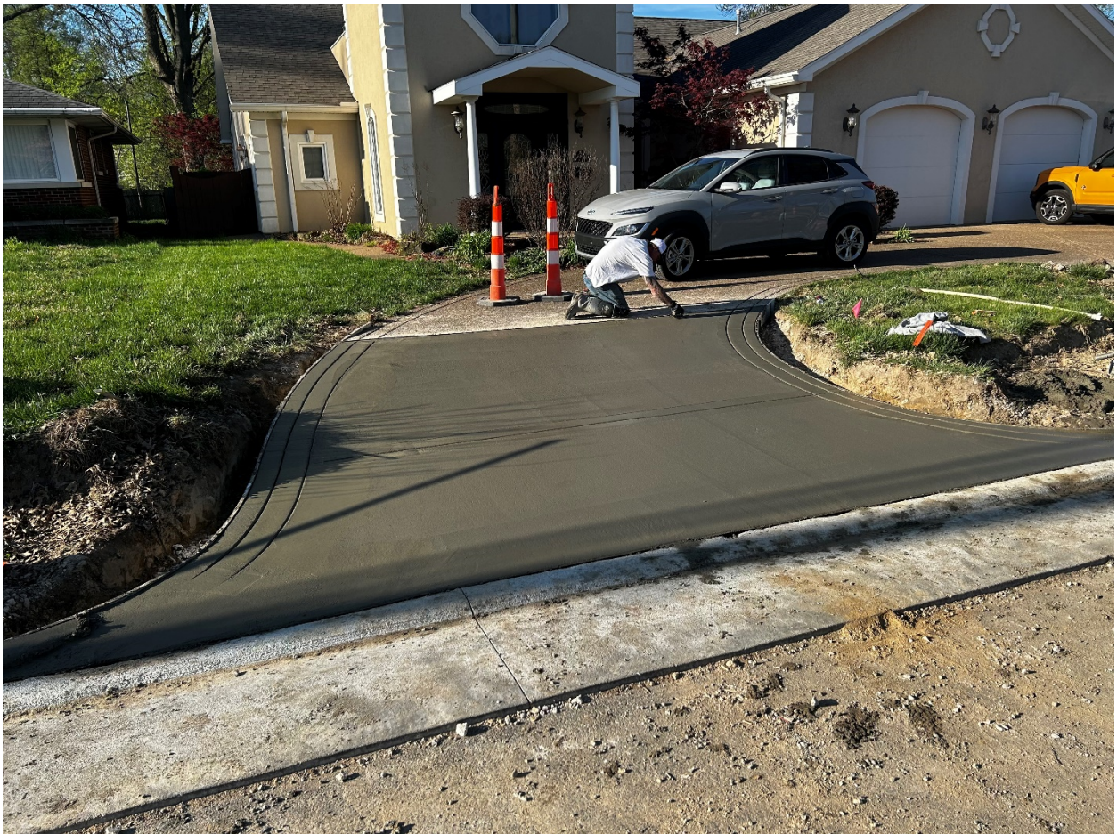
(BBI finishing the exposed aggregate drive approach at 2061 E Walnut Street.)
