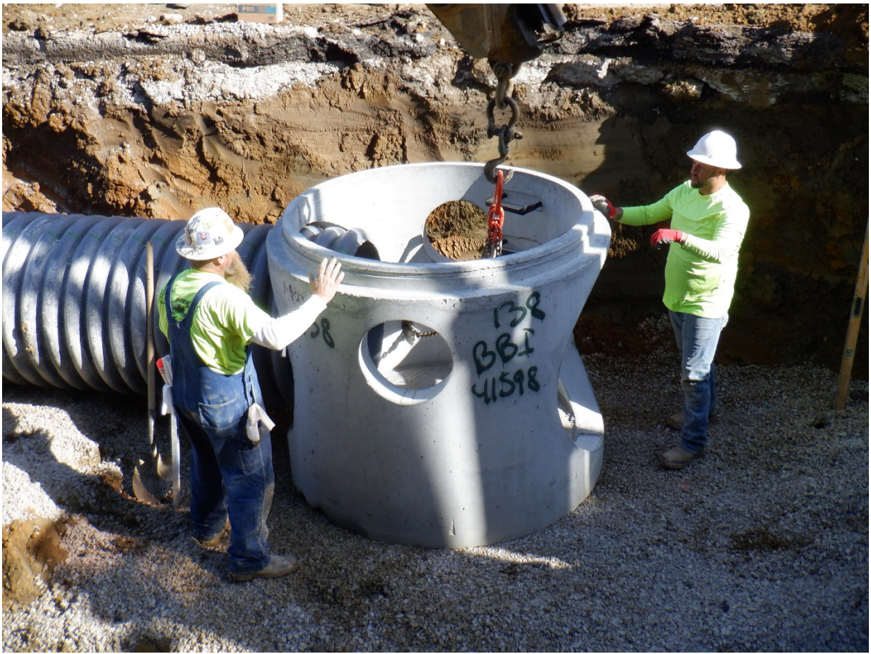
(BBI installing 36" storm sewer and Manhole Str. #138 along Walnut Street.)
