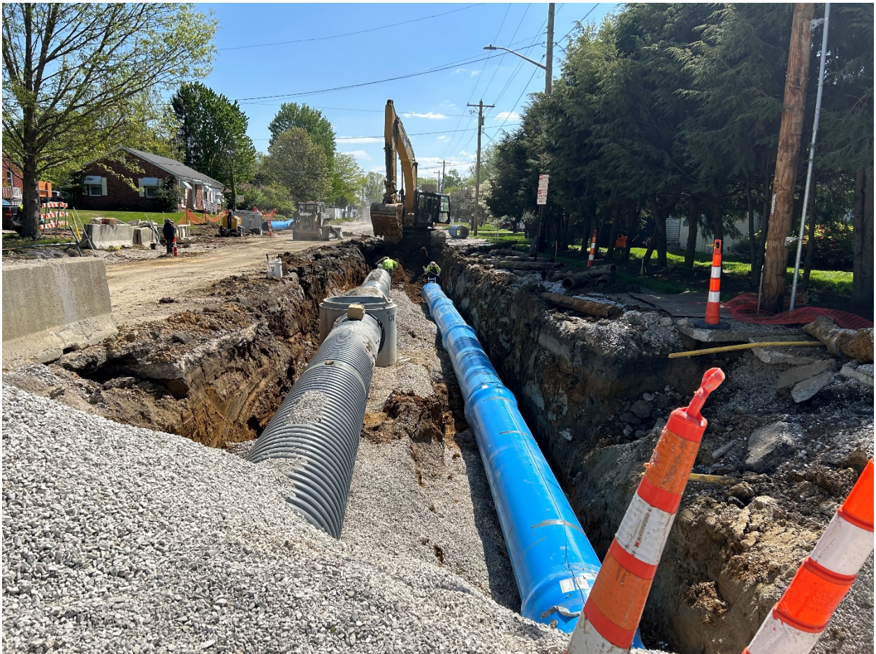
(BBI installing 36" storm sewer and 30" force main along Walnut Street.)
