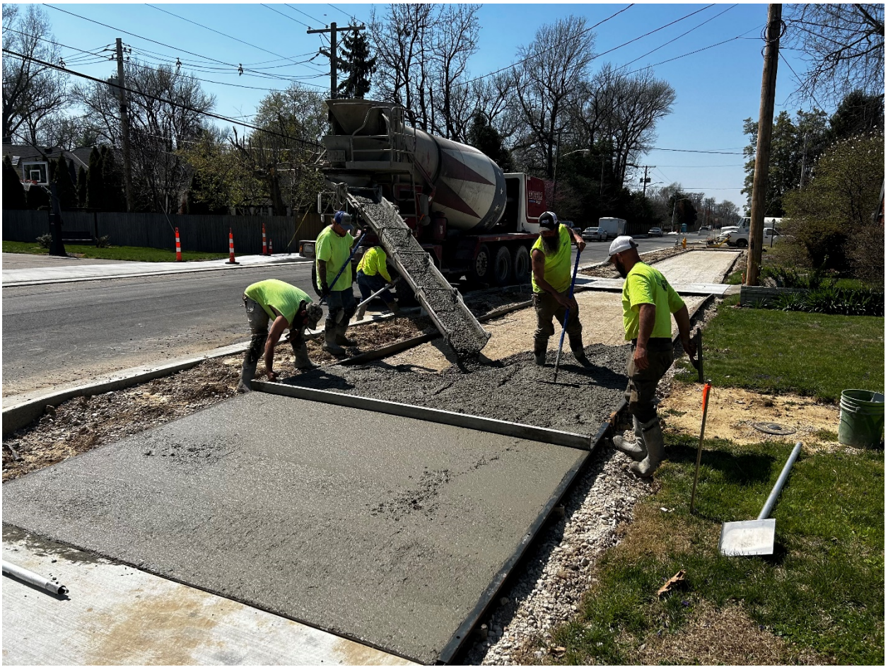
(BBI pouring multi-use trail along the north side of Walnut Street.)
